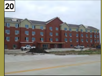
Townplace Suites by Marriott 1832 Marketplace Drive Valuation: $3 million Permit Issuance: April 2013
