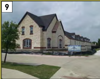
9 Out of Space Storage 3920 S. Ridge Rd. Valuation: $3 million Permit Issuance: October 2014
