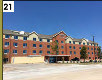
21 Townplace Suites by Marriott 1832 Marketplace Drive Valuation: $3 million Permit Issuance: April 2013
