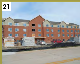
Townplace Suites by Marriott 1832 Marketplace Drive Valuation: $3 million Permit Issuance: April 2013
