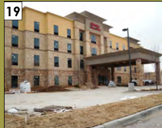
Hampton Inn & Suites 2008 N. Central Expressway Valuation: $3.5 million Permit Issuance: Jan 2014
