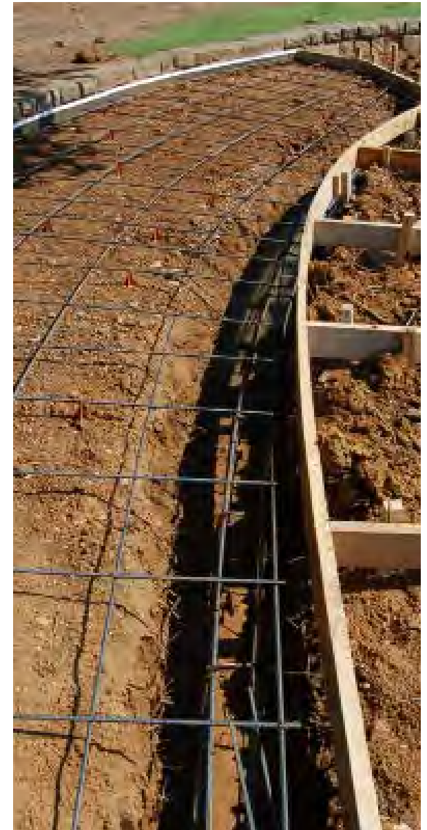
Trail Under Construction
